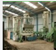
Shredder residue treatment
